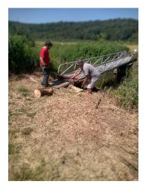
One of the metal bridges crossing the ditch in the field was not level. This was corrected by leveling and securing the bases at each side of the bridge using some "good ole VT" leverage work to raise the bridge so work could be done on the base.
